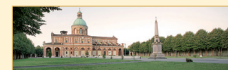
The monumental shrine rises at the center of a vast oplanado surrounded by symmetrical porticos on all four sides, that run with 200 arches for almost 600 meters
